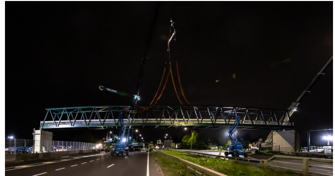
The footbridge being lifted into place
