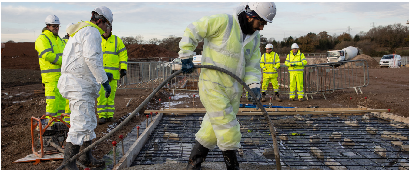
On-site trials of low-carbon concrete
